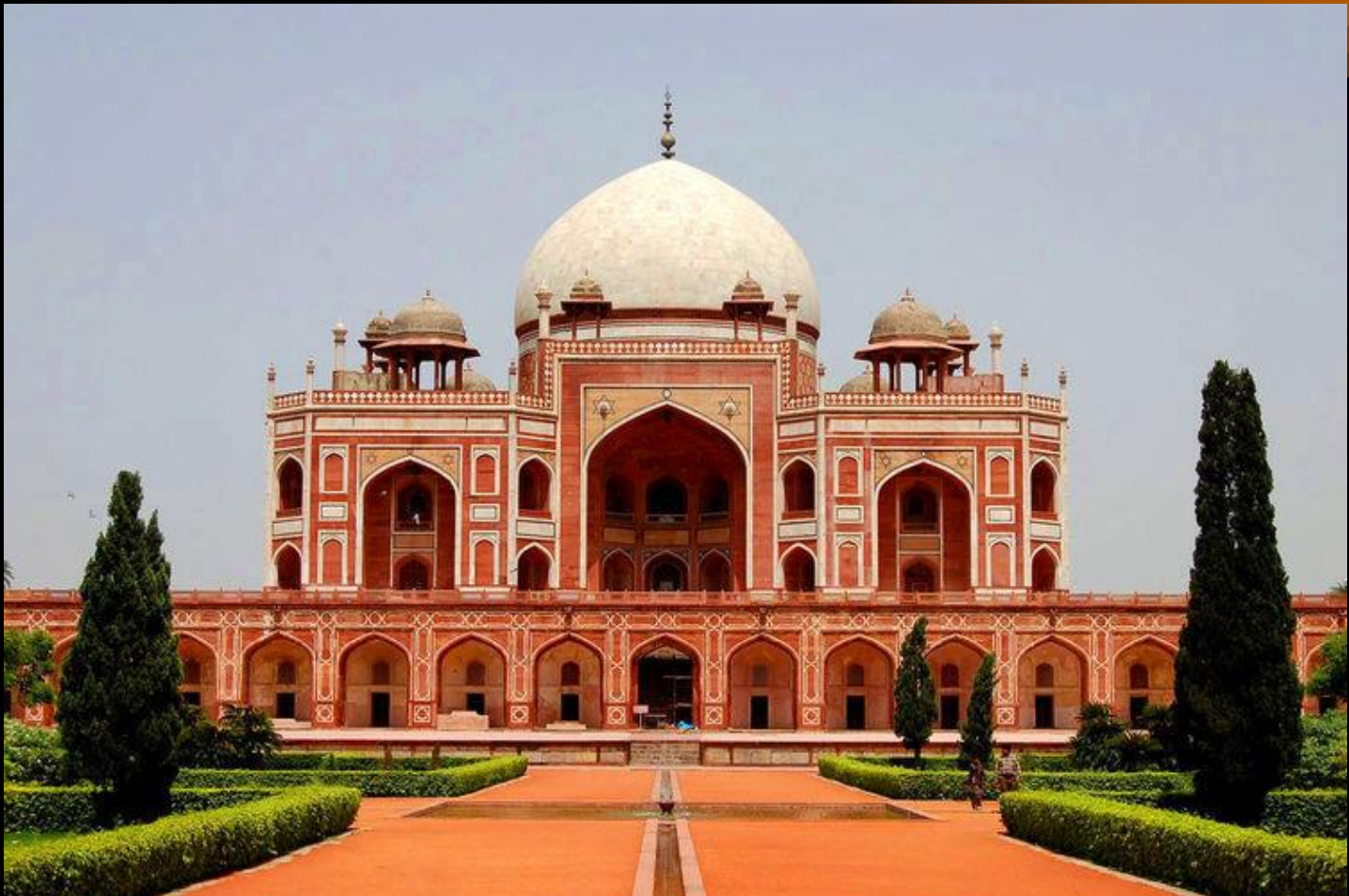
Akbar's Architecture : Plain dome
